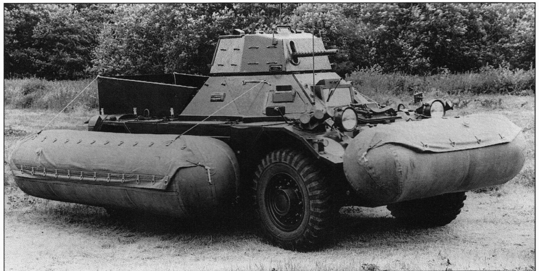
Top right. Prototype number 5 of the Swingfire-equipped Mk 5 variant undergoing so-called trundling trials during 1967. This is yet another conversion, unfortunately of uncertain parentage. Compare the shape of the stowage bin for the reload-missiles with those on the mock-up shown opposite. (TMB, 2058 C1)
